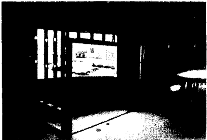
Fig. 12 — Balconies were formed by framing off portion of interior circular silo space.
