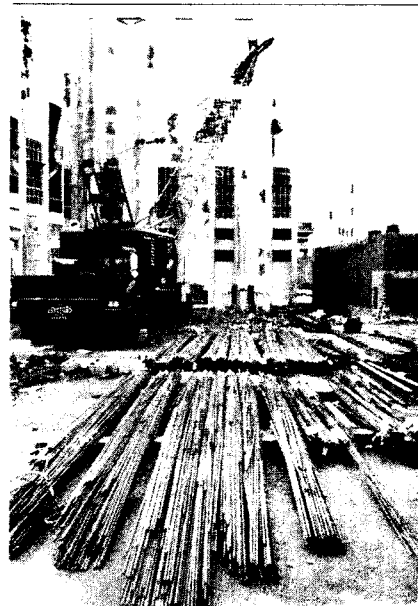
Fig. 10 — Foreground: Stockpiled No. 5 reinforcing bars for floor slab construction. Background: Worker prepares sawcut silo wall section for removal.
