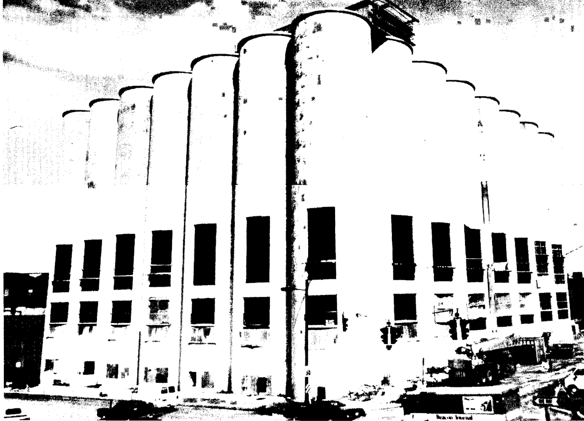
Fig. 1 — Quaker Square Hilton under construction. The L-shaped complex of 36 concrete silos was reconstructed to form a first-class convention hotel.
