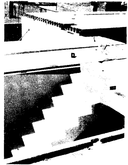
Fig. 6 — Precast concrete stairs.
