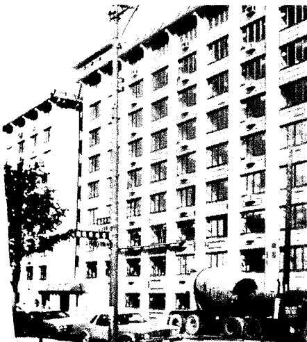
Fig. 3 — The 9-story, wall bearing low-rise was built in busy, congested Chicago's Chinatown.
