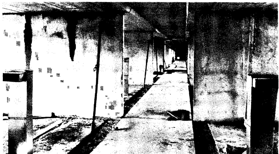
Fig. 4 — Precast 6 in. (152 mm) thick concrete load-bearing walls were braced until they reached sufficient strength.
